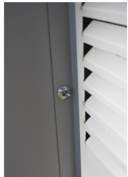
Step 21 screw in fixing bolts to connect heat pump module to storage tank
