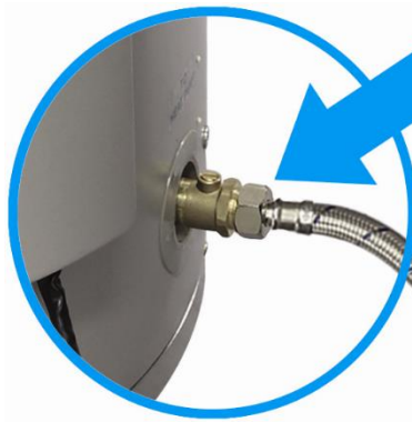
Step 13 attach flexible hose with blue stripe to inlet and ball valve in open position
