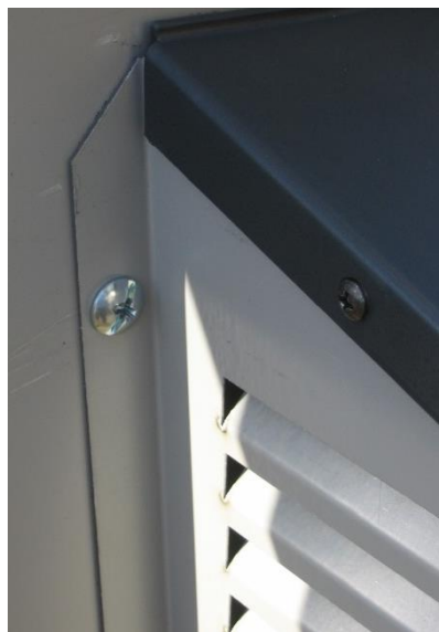
Step 21 screw in fixing bolts to connect heat pump module to storage tank
