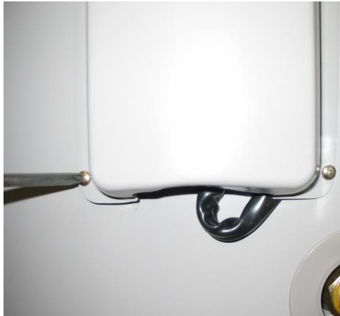
Step 2 remove screws from lower front cover
